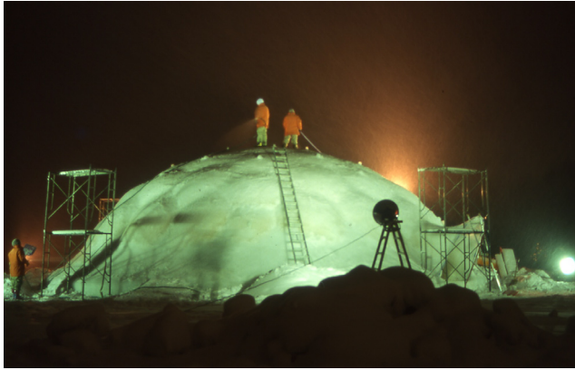
Fig.2 Spraying water on ice dome under construction
