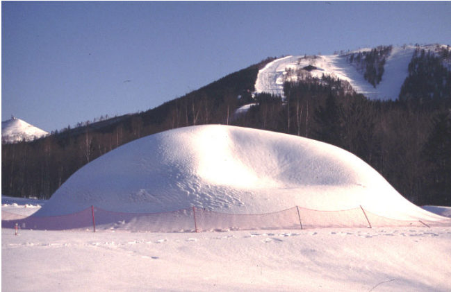
Fig. 5 Large creep deformation before collapse
