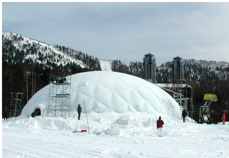
(b) Construction of 30m ice dome(Base diameter=25.0m, Height=9.2m)
