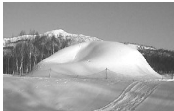
Fig.11 Large deformation right before collapse
