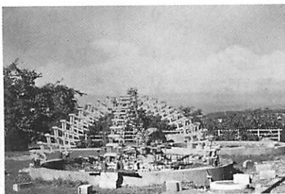
Fig.10 Lifting up (wooden dome)
